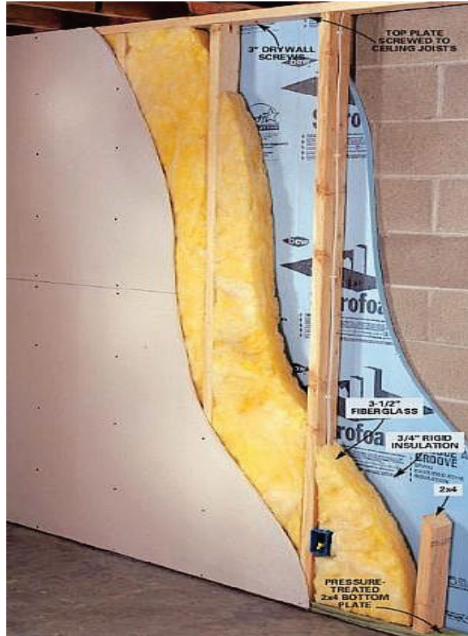
Figure 3-32: Masonry Wall With Furring Details
