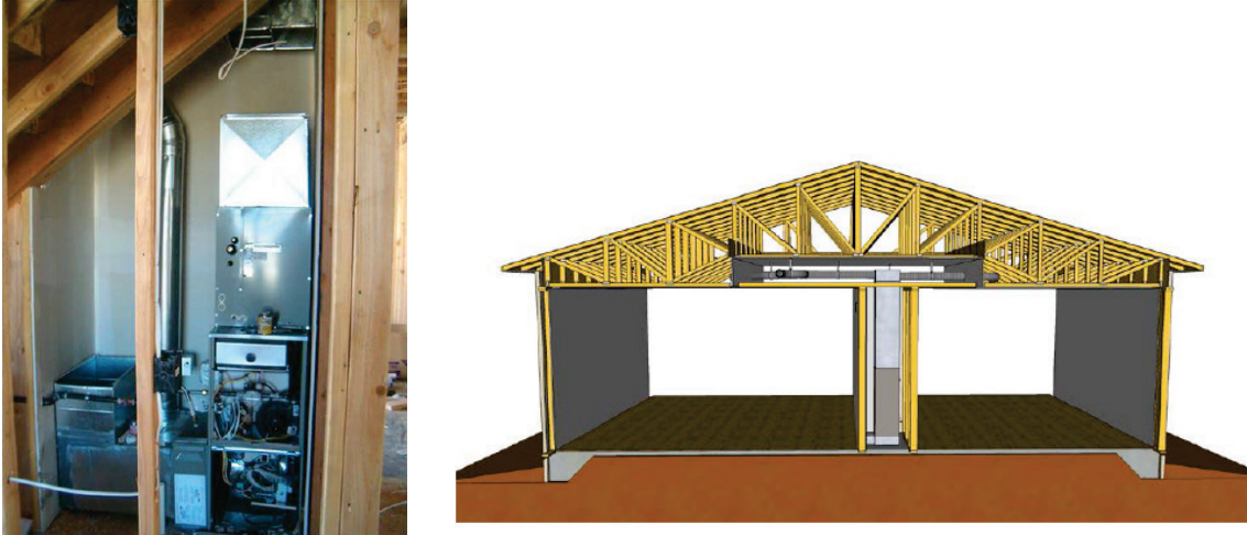
Figure 4-14: Mechanical Closet Placement Example
