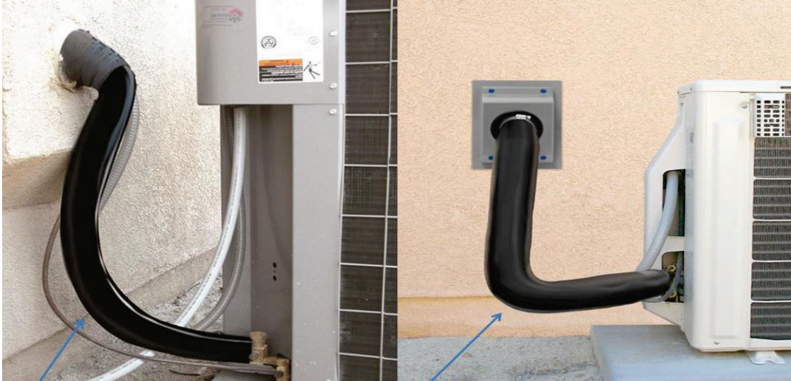
Figure 4-1: Refrigerant Line Insulation
