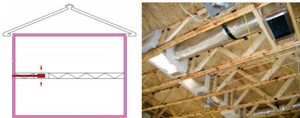
Figure 4-13: Open Web Floor Truss Example
