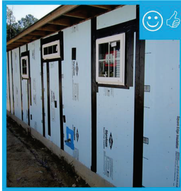
Figure 3-53: Properly Installed Rigid Insulation With Sealant Tape
